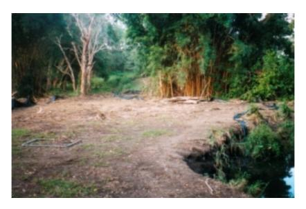
Examination shows the silt barriers rendered completely useless, the bank vegetation stripped, the bank unprotected, trees removed and all built up debris, which provides both surface protection and habitat, stripped.
