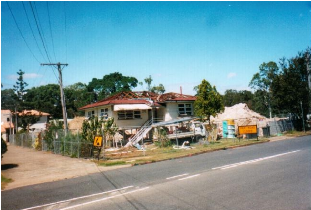
An example where demolition allegedly preceded approval for development.
