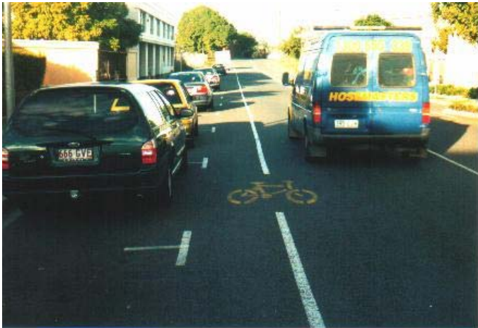
Figure 7. Marked car parking bays keep vehicles parked close to the kerb.
