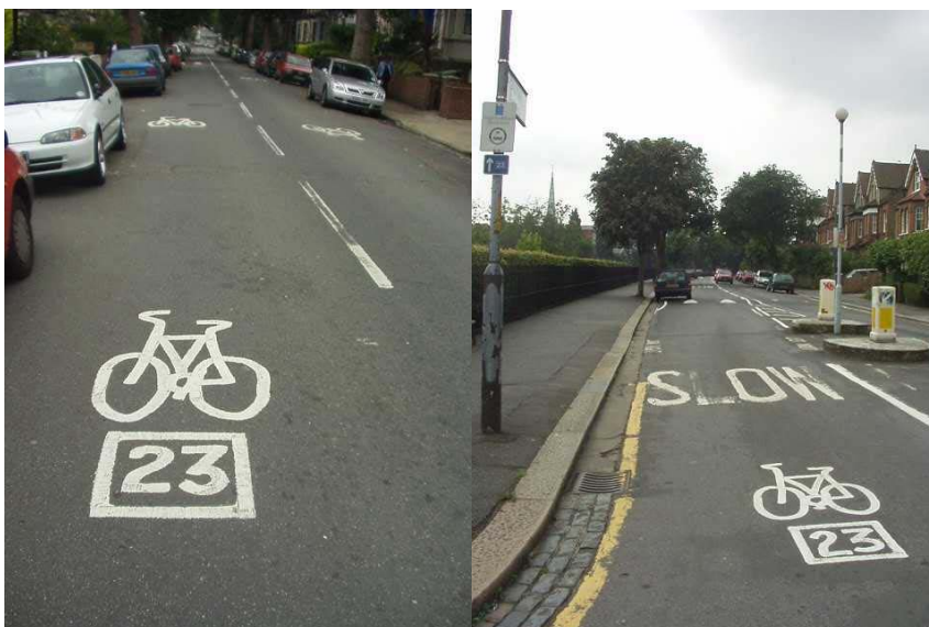
Figures 5 and 6. Shared lane symbol on London Cycle Network route 23 in Southwark.
